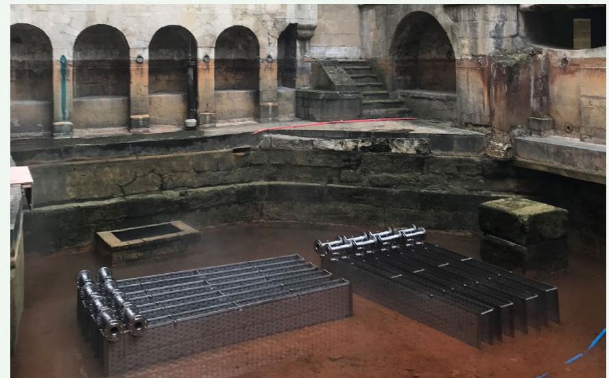
King's Bath drained with energy blades
